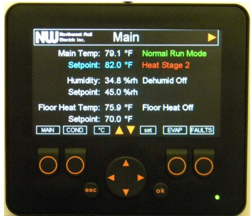
Main HVAC system display screen (above) and a small portion of the technical details and system status and fault monitoring that is available (below). System includes detail displays for condenser and evaporator status and many other items helpful for diagnosis.
