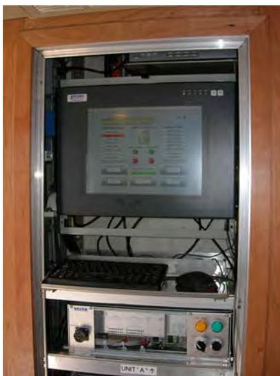
Connection schemes, display and control systems (touch screen, switch, button, or keyboard and mouse), and enclosure type are all selected to suit the needs of the customer.
