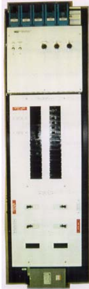
HVAC Control, Emergency Lights, and Circuit Breakers
